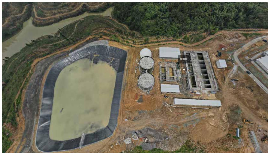
The waste treatment system of a complex of pig buildings.
