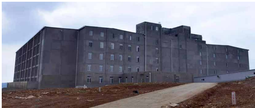
A multi-level pig building can be a complete ‘all-in-one’ integrated pig production chain with a sow unit, nursing and fattening areas.
